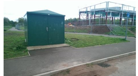
Refurbishment of 2 old WPD subs
