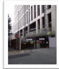
Carillion, One St.Peters
