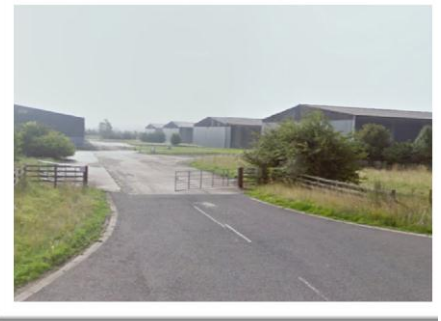
Mid UK Recycling Centre in Ancaster, Caythorpe, with 10,000 m cable route to WPD Primary Substation
